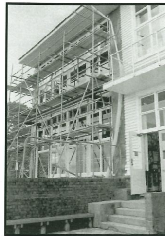
Two new classrooms in the two-storey block, opened July 2000.
