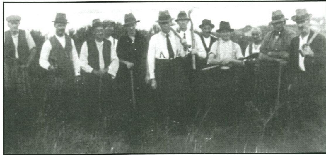
Clearing the land, 1925.
